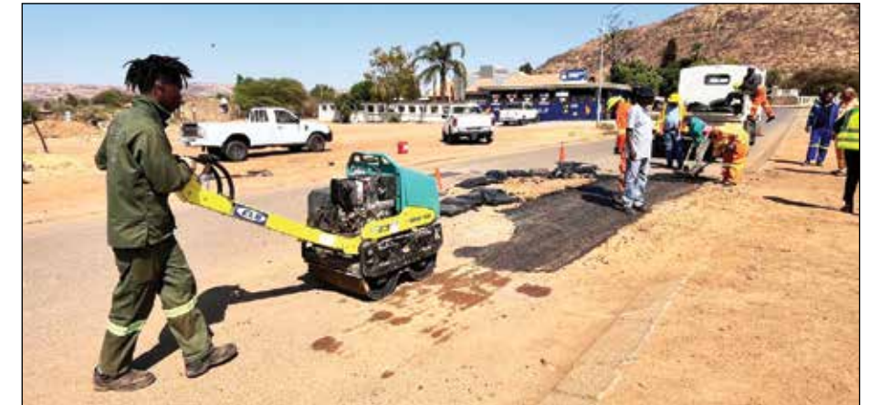
Patching of potholes at Mabele-A-Pudi village in the Moses Kotane Local Municipality as part of the Accelerated Service Delivery Programme - Thuntsha Lerole
